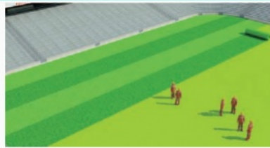
3. Artificial turf laying process
