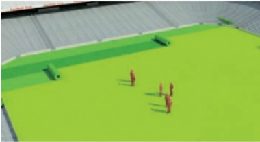
2. Laying of artificial turf
