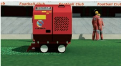
6. Installing the infill granule
