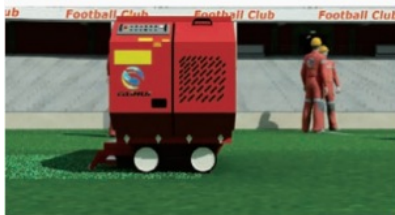
6. Installing the infill granule
