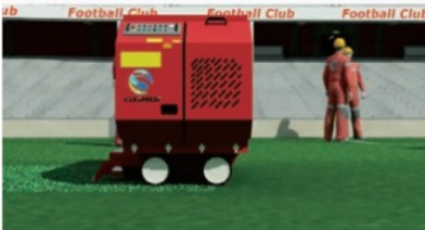
6. Installing the infill granule
